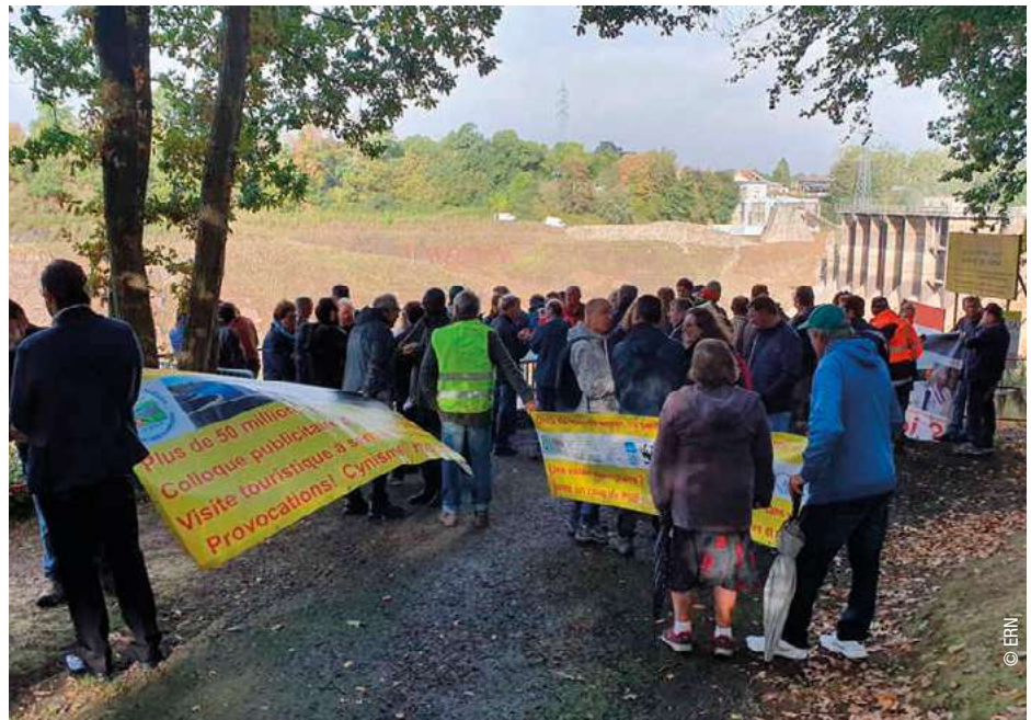
The visit to the dam-removal worksite in Vezins (Manche department) on the Sélune River, on 26 September 2019.
